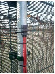
Illustration of Seismics Sensors deployed along the border as a part or Early Warning
