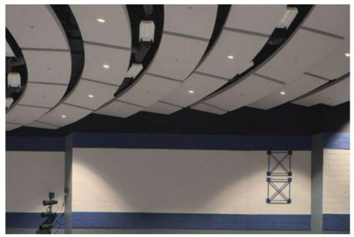
Usage of Ceiling & Wall Panels of Different Material Finishes to Match Décor Seamless Gloss Absorptive Ceiling Treatments – ABSORPTION
