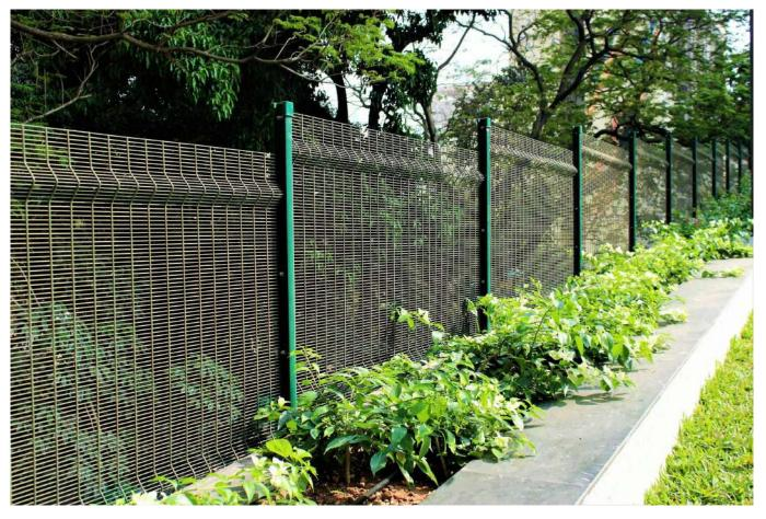
Weldmesh is finding increasing use for securing not just borders but also our regular assets like commercial, residential, industrial and institutional buildings. The advantages of welded mesh as an alternative to chainlink fence has resulted in its fast acceptance in the market, despite being slightly expensive on account of using more steel. Some of the key advantages are:
